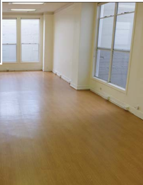
The finished floor gleams in the Office of Self-Help's multipurpose room at 944 Market St. Inset: Welker Bros. installer levels the floor before laying the vinyl.
