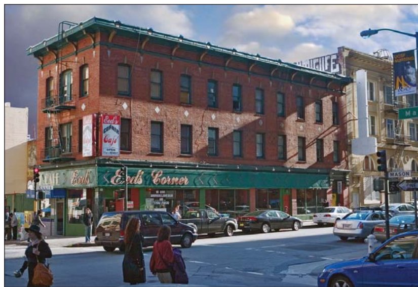
Ed's Corner anchors 201-31 Ellis St., which also houses Thai Noodle Café and Hostel and Hamman Sultan Baths. The building was built in 1910, architect Smith O'Brien.
